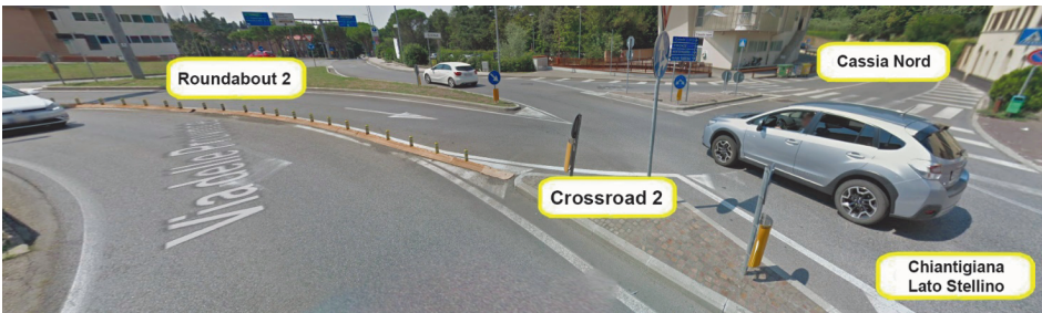
Figure 5. Crossroad 2 view from Chiantigiana Lato Stellino
