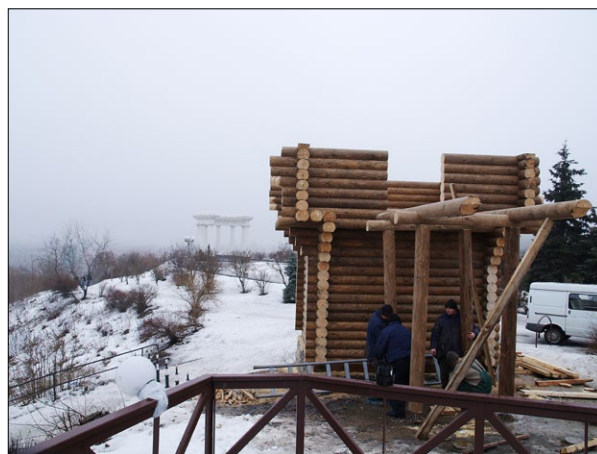
Fig. 7. Construction of the Podilska tower, February 06, 2009; photo by K.Y. Trehubov.
