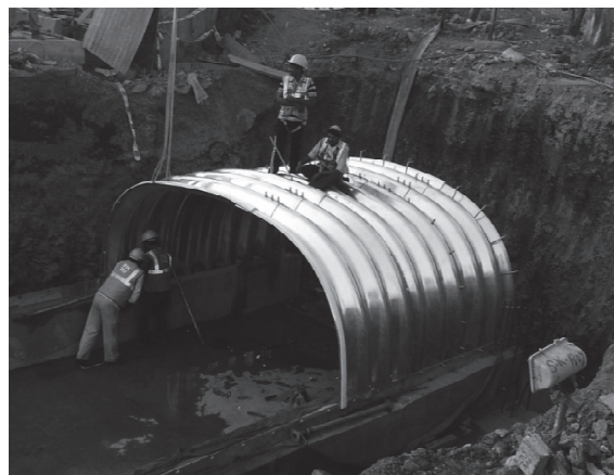
Fig. 4. Installation in progress
