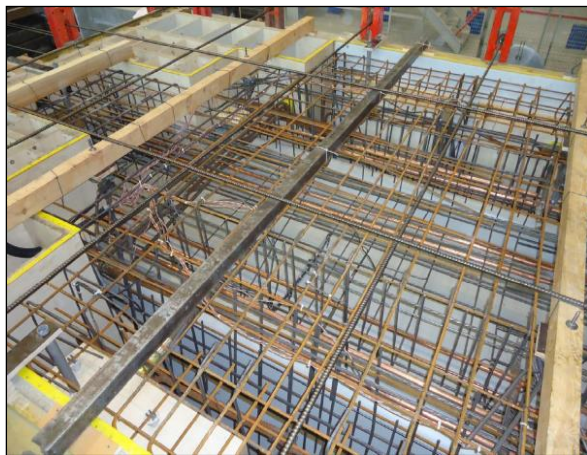
Fig. 10. Steel reinforcement in concrete
