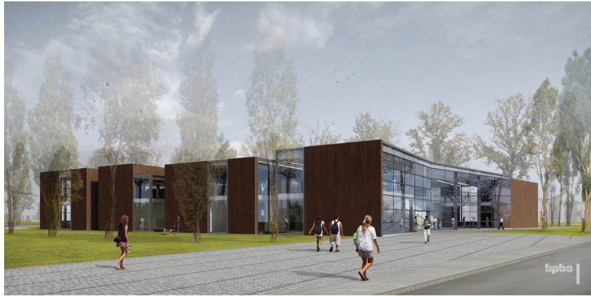
Fig. 2. Visualisation "View from the southeast"; Provided by the director of Mediatheque, Mrs. Renata Wojtczak
