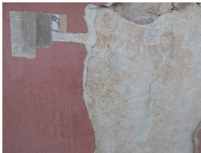
Fig. 3. Sounding of painting layers of the façade in 28, Market Square (the second floor). The first layer of paint was light ochre (ivory) color similar to the sandstone color. Source: photo by author
