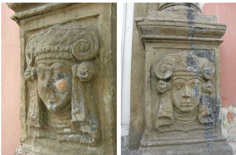
Fig. 7. The soundings of the authentic polychromy of the sandstone details (28, Market Square) – the orange paint on the mask (the 1 st period of polychromy) and complete black painting (the 2 nd period of polychromy). Source: photo by author
