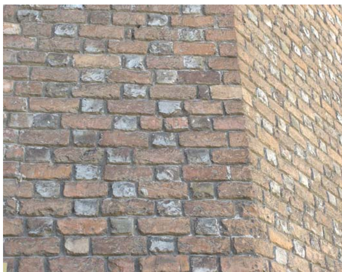
Fig. 1. The Gothic bonding with strongly baked heads (the Tower near City Arsenal). Source: photo by author
