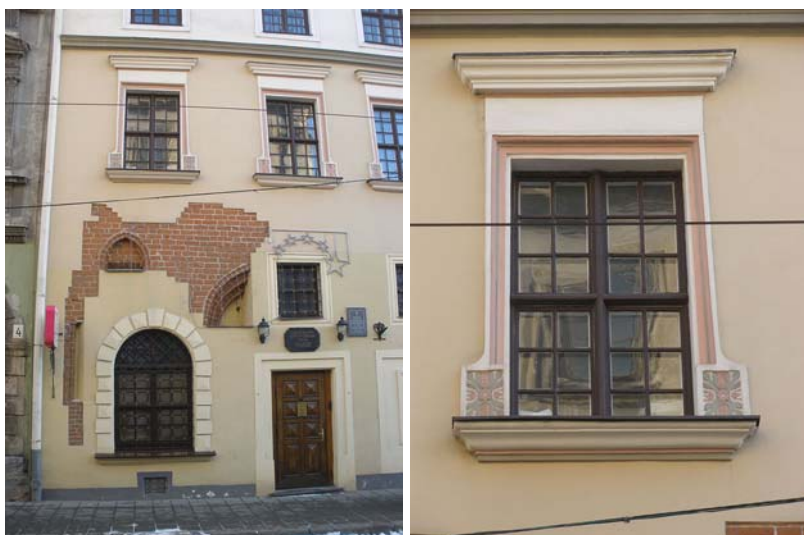
Fig. 2. Restoration of the renaissance façade polychromy with the sounding of gothic brick masonry (2, Ruska Str.) Source: photos by author
