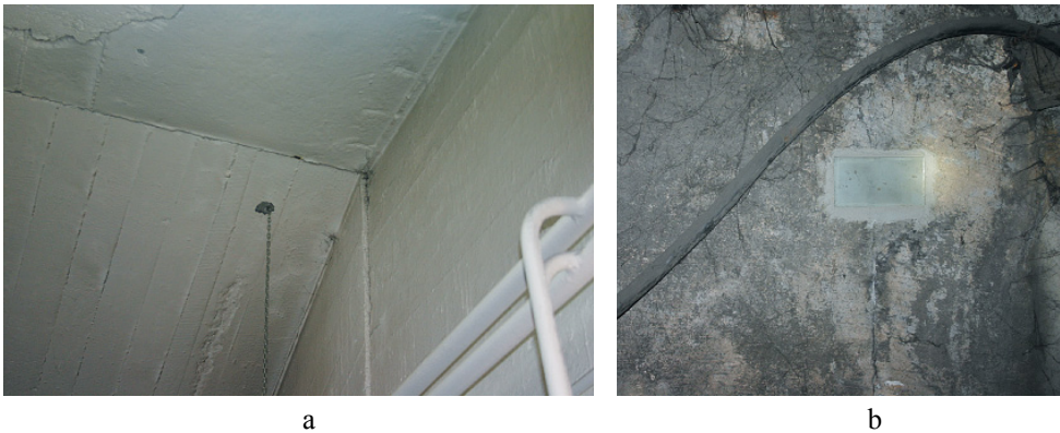
Fig. 3. Recorded damage a) displacement of ventilation head, b) view of the installed seal
