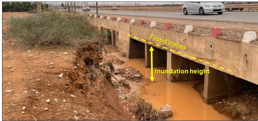
Figure 11. Inundation height in the intersection of national road N2 and Sefrou wadi
