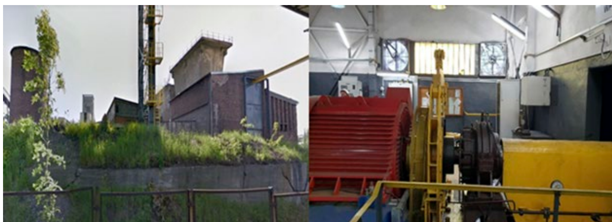
Figure 1. Main fan station of mine Y
