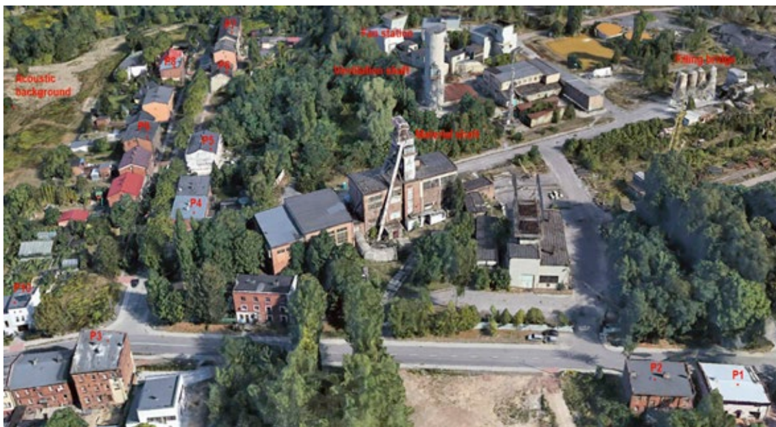
Figure 4. Location of measuring points around the fan station of mine Y
