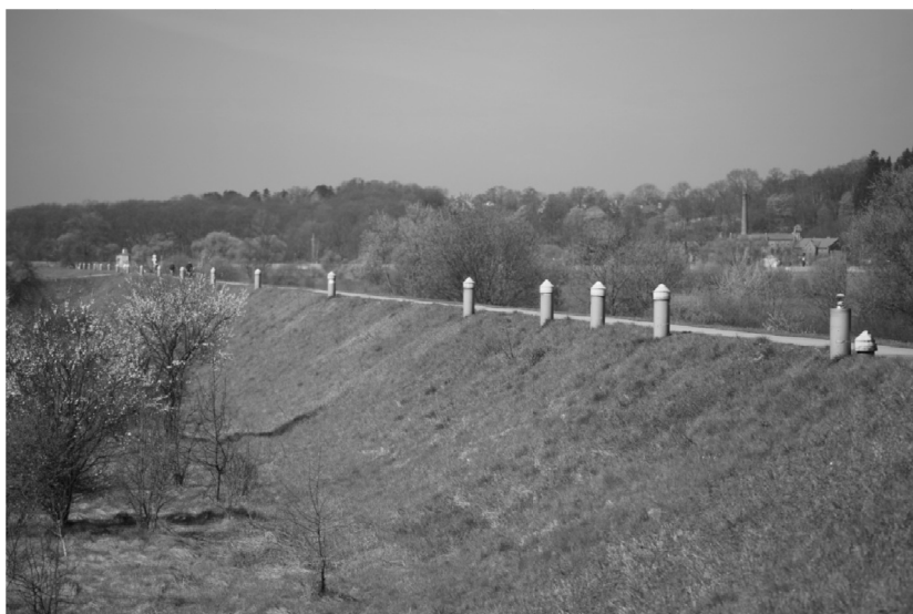
Fig. 1. „Wisła” testing baseline – view from point „0” toward the E direction.
