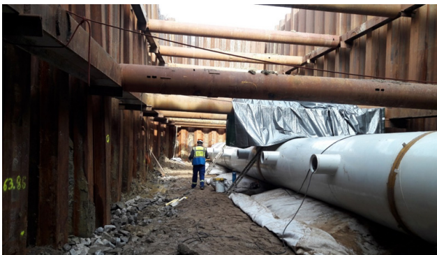
Figure 3: The discharge system during construction.
