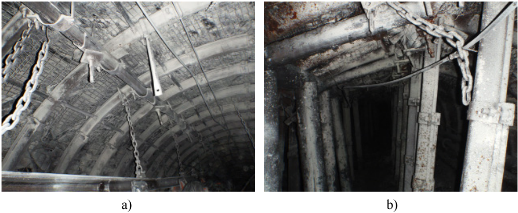
Fig. 1. Examples of a gateroad support where underground measurements of deformation were conducted, a – yielding steel arches, reinforced with steel horseheads bolted with flexible bolts view of the gateroad ahead of the longwall face, b – yielding steel arches, reinforced with wooden and steel props, view of the gateroad behind the longwall face
