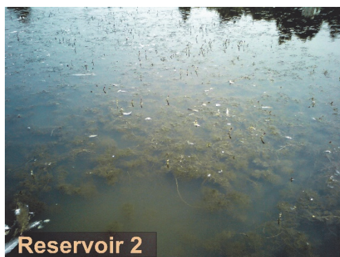
Fig. 5. Intensive plant development on the sealed bottom of reservoir
