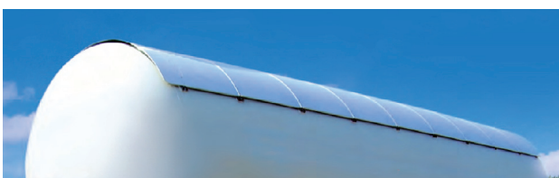
Fig. 6. A sun shield covering the top part of a tank [1]
