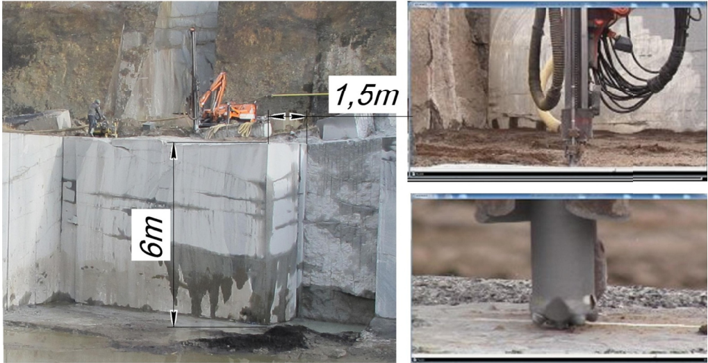
Fig. 2. Timing of borehole drilling by a drilling machine COMANDO 110
