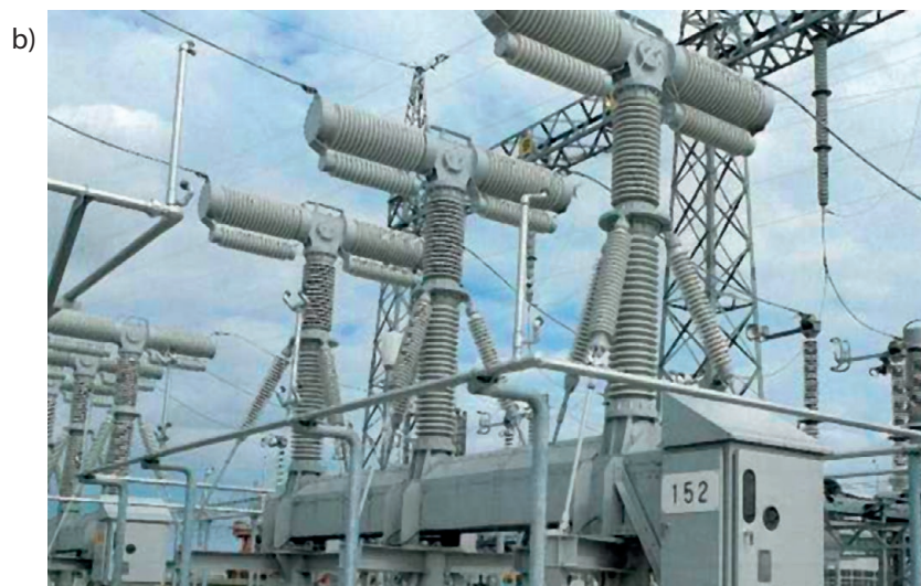
Design: live tank Rated voltage: 168 kV Rated current: 2,000 A Short-circuit current: 31.5 kA Additional insulation: SF 6 No. of vacuum chambers: 2/phase Mechanism: spring-stored energy
