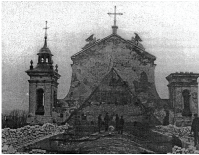
Fig. 10. View of the vault of the main nave walls after the failure associated with the collapse of the structure of the roof due to a fire that occurred in the past.
