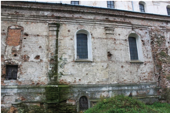
Fig. 8 View of the facade from the eastern side of the building,
