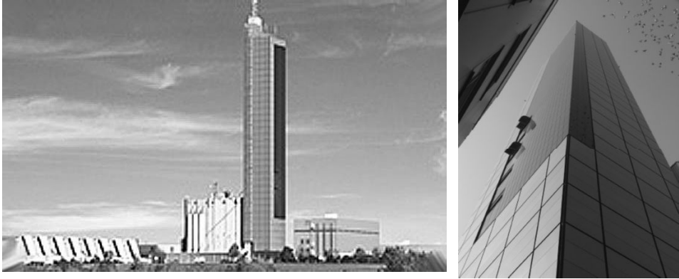
Fig. 9. Grain silo in Ulm including the PV installation [23, 27, 30]
