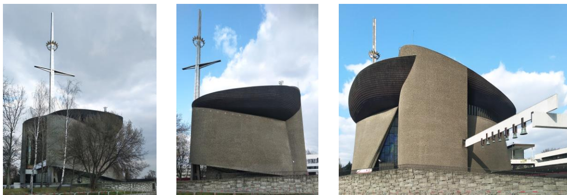
Fig. 7-9. The first church of Our Lady, The Queen of Poland, in Kraków - Nowa Huta (W. Pietrzyk; under construction in 1967-1977). Source: Photo courtesy of the Author
