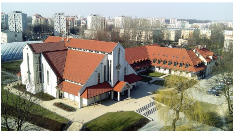
Fig. 16-17. Working model and a view of the entire parish complex in Kraków - Nowa Huta, following its completion. Source: Reproduction and photo courtesy of the Author
