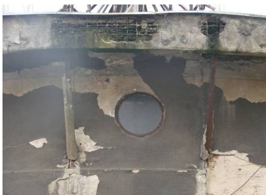
Fig. 5. Metal window opening, 2017. Source: author Ryc. 5. A metal window opening of a degraded water tower, 2017r. Źródło: autor
