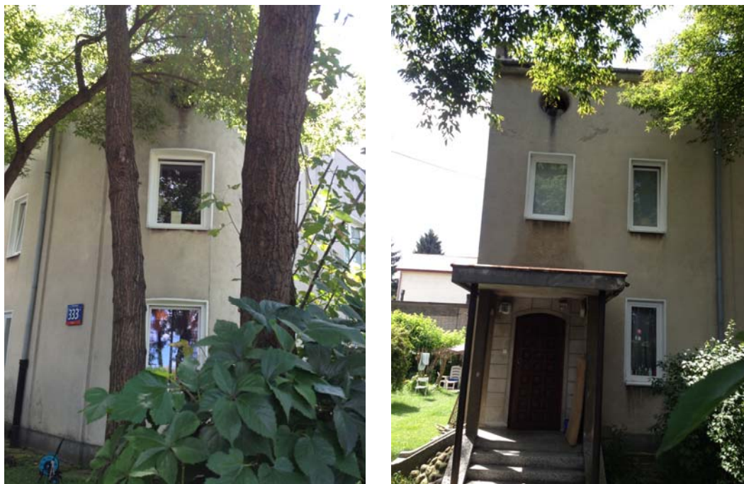
Fig. 2. i Fig. 3. Detached house at Wilanowska 333, Warsaw, included in local register of monuments, photo: R. Barełkowski, 2014.
