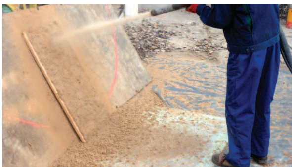
Photo 2. Application of the selected plaster onto substrate made of OSB panels
