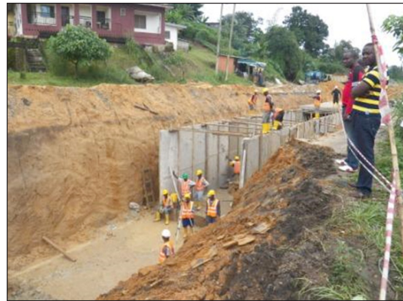
Figure 4. An underground canal under construction in Calabar (Photo by authors)
