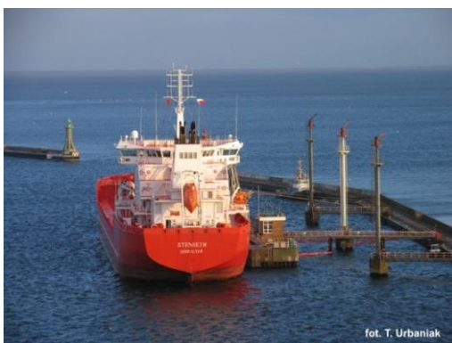
Figure 2. Fuel Reloading Post in Gdynia Port
