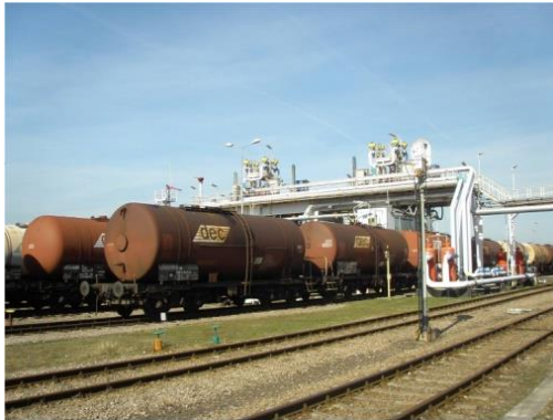
Figure 5. On-spot loading device in Part C
