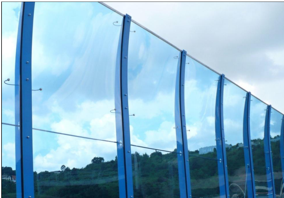
Fig. 5. Reflective surface noise barrier [13].
