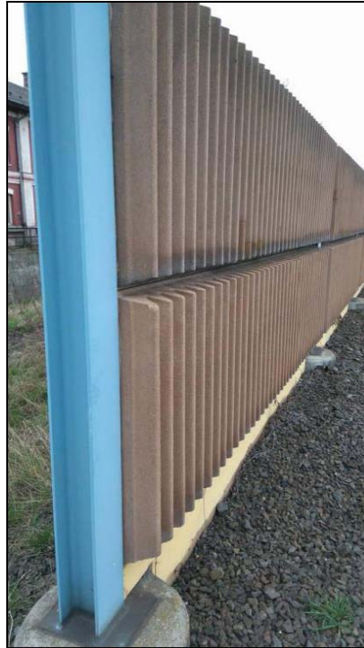
Fig. 6. The surface of the absorptive noise barrier [13].
