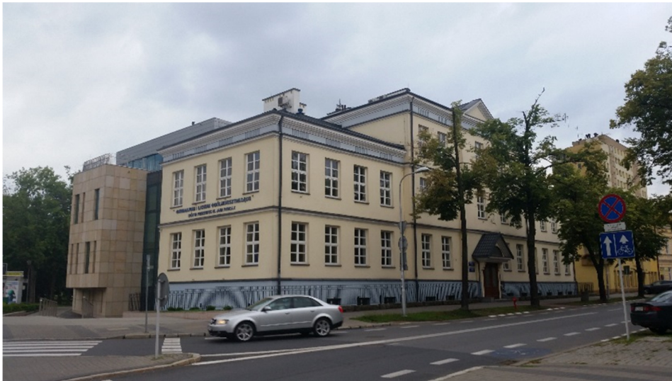
Fig. 1. View on the analyzed building with extended part
