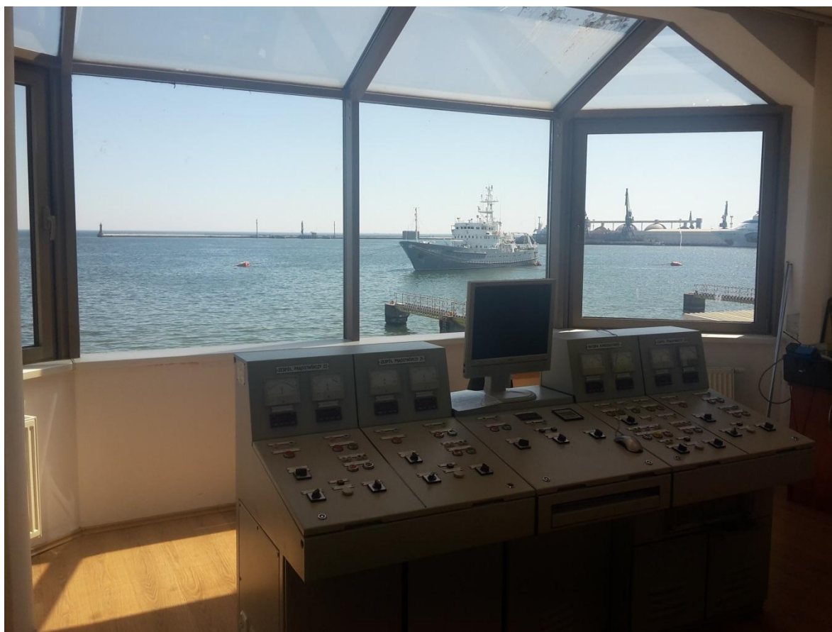
Fig. 4. View of the operator console at the new Coastal Station of Demagnetization of Ships, 2017. Photo by K. Kaminska.
