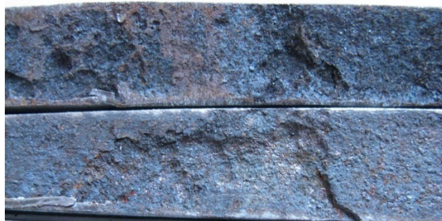
Fig. 1. General view of the inner wall of the pipe
