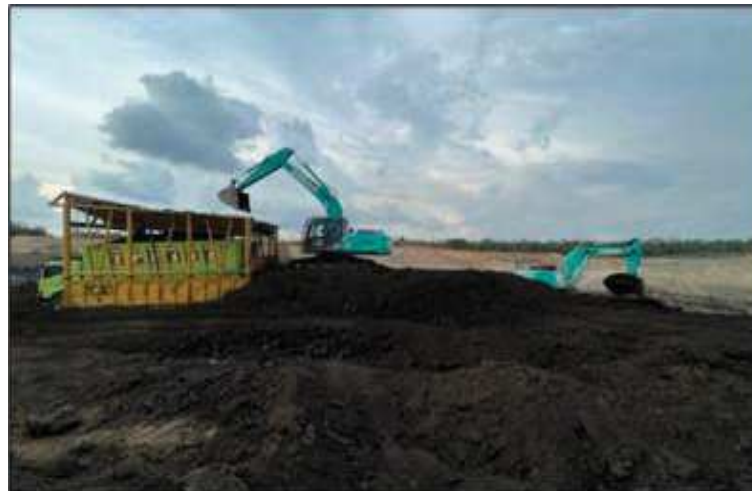
Fig. 4. Coal Extraction with In-pit Processing
