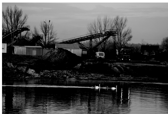
Fig. 5. Sand and gravel mining in the Raba River Valley. Targowisko-Zakole locality near Klaj (photo by: A. Kowalska)
