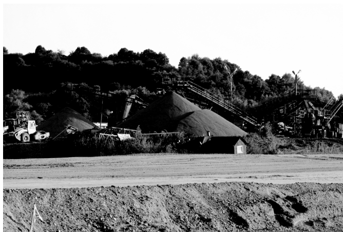
Fig. 4. Gravel mine in Klaj. In the foreground: construction works on new motorway in progress (photo by: A. Kowalska)
