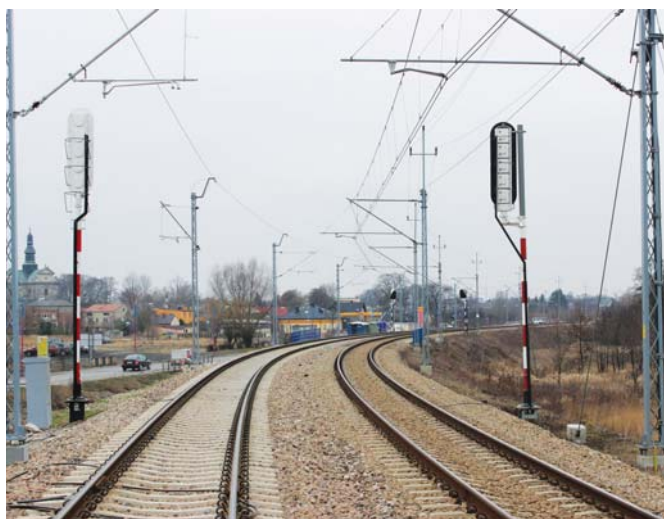
Revitalised section of line No 61 at Koniecpol
