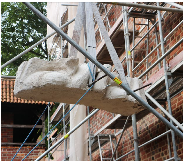
Fig. 9. Transport of the finished segments of the Madonna statue to its place in the outer niche of the presbytery, 2015; photo by L. Okoński.
