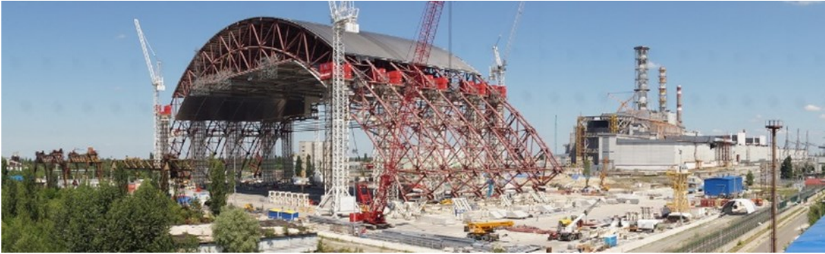
Fig. 2. NSC after second lift of eastern section in 2013.
