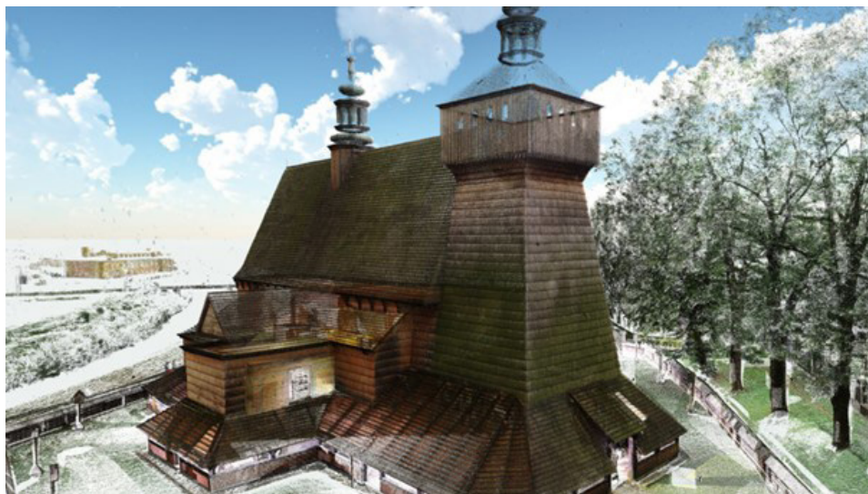
Fig. 2 Point-cloud with texture depicting the church from the north-west (image by Wojciech Markowski)
