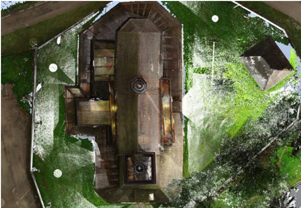
Fig. 6. The point-cloud with texture depicting the roofs of the church (image by Wojciech Markowski)
