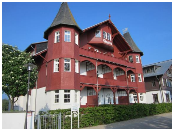
Fig. 17. Bansin, Prefabricated Villa Vineta and Villa Strandklause by Wolgaster Holzbau. Source: Wikimedia Commons
