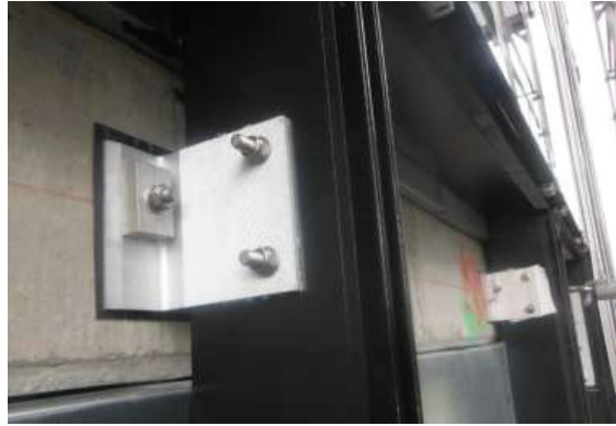
Fig. 1. View on fixed aluminium brackets in mullion-transom wall system
