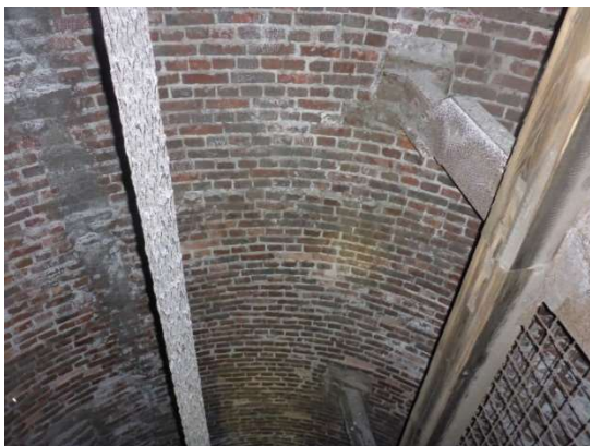
Fig. 2 Lining of shaft X at the depth of about 300 m
