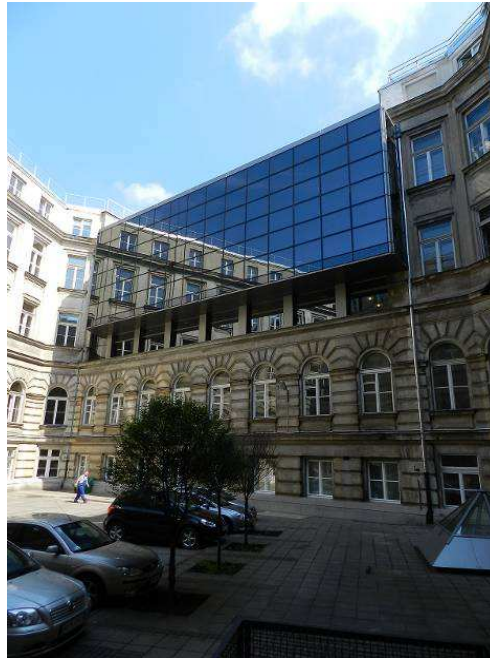
Fig. 2. Main Building. Internal view with super-structured library in 1996-1998.
