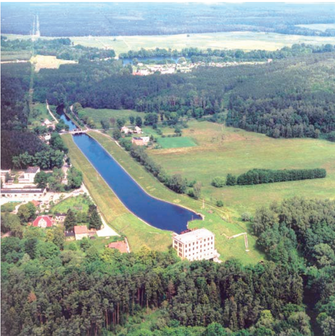
Fig. 3. View to Gródek hydroelectric plant with inlet channel
