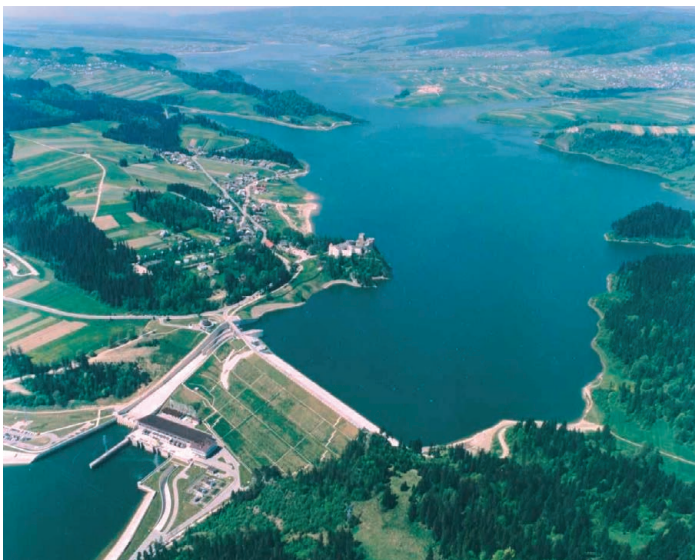
Fig. 8. View of Czorsztyn-Niedzica dam, with surface overflow and power plant, and with reservoir
