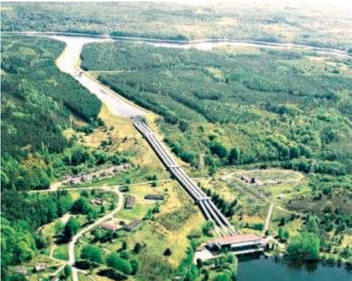
Fig. 9. View of Żydowo hydropower plant and its open channel and pipelines
