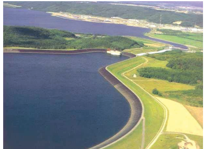
Fig. 10. View of the upper reservoir of the pumped-storage power plant, pipelines, and Lake Żarnowieckie
