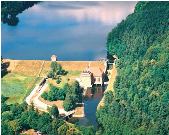
Fig. 1. Łapino hydropower plant in the Radunia River
