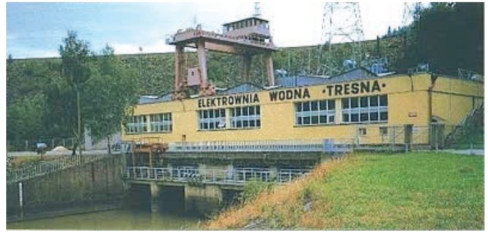
Fig. 6. View from Tresna hydropower plant's tail water, with earth dam in the background
