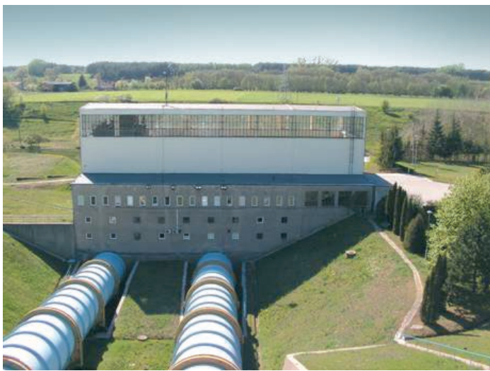
Fig. 5. Koronowo hydropower plant. View of two pipelines supplying water to the plant
