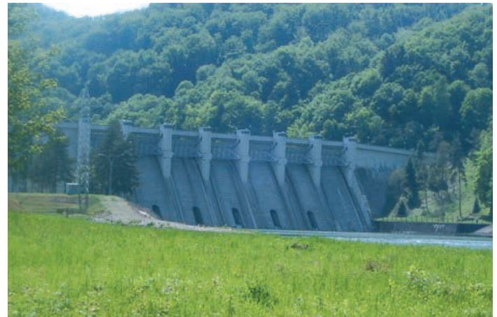
Fig. 4. View to Rożnów dam from the tail water. Visible spillways closed with segments, and bottom outlets
