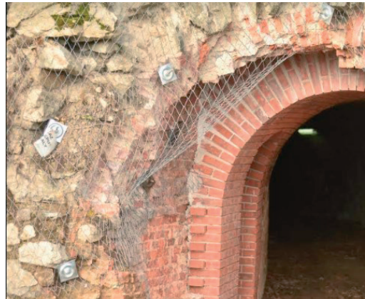
Photo 9. Protection of the damaged wall's face with a steel mesh mounted by the anchors (photographer – Grzegorz Basiński)
