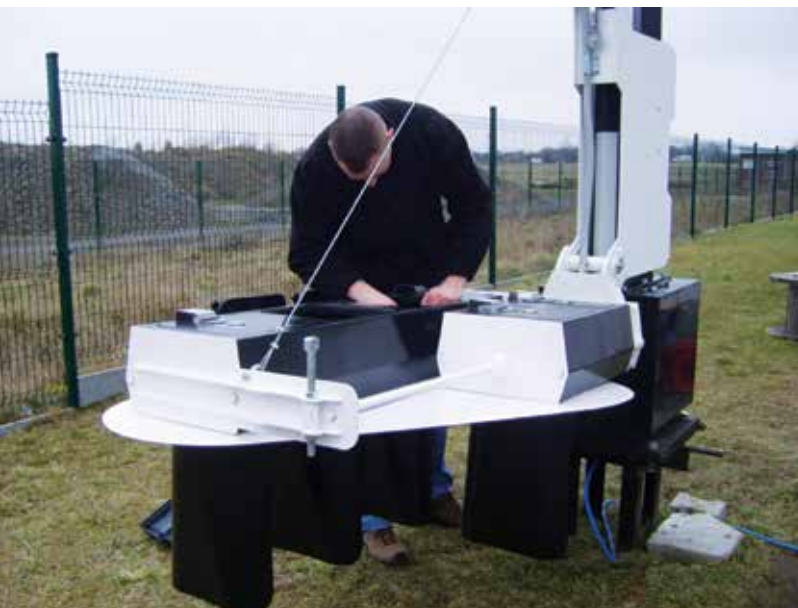
Maintenance works on the signal with movable head
