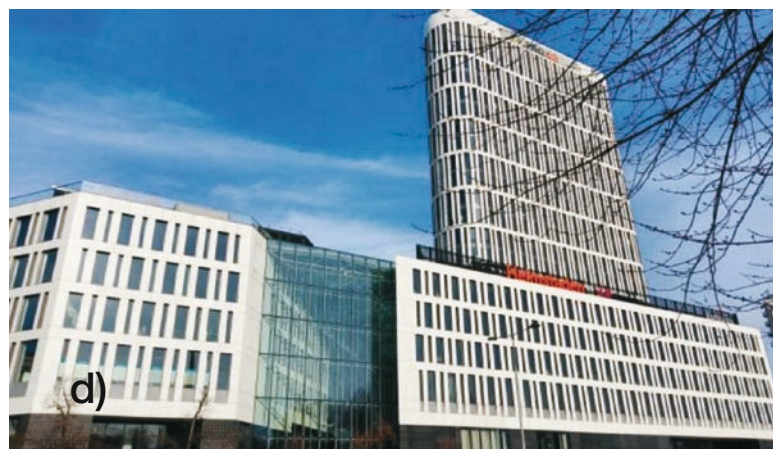
Fig. 2a-d. Plac Unii building, Warsaw, APA Kuryłowicz; source: photo by the author (2023).
