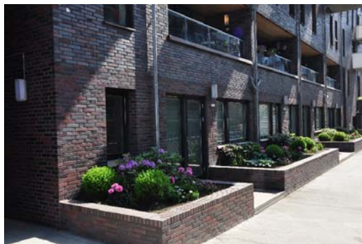
Fig. 1 B Living estate with ground floor flats with tiny front gardens in Oslo (Norway). Source: author's photo
