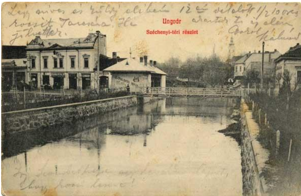
Fig. 7. Small Uzh already during the formation of the flow [10]
