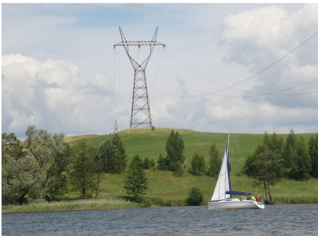
Fig. 1. An overhead power transmission line - Tałty Lake. Source: W. Gadomska
