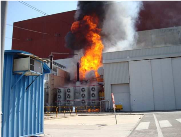
Figure 6. Development of fire in a transformer
