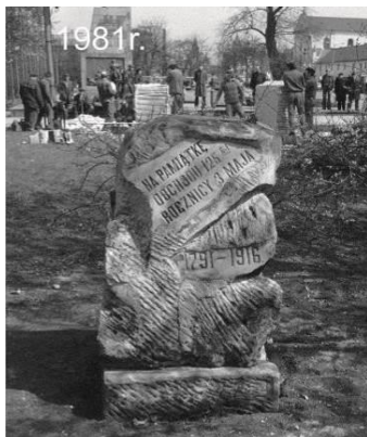
Fig. 11. Monument to the May 3 Constitution after renovation in 1981, prepared for once again being placed in the square in its southwestern corner. Source: Archive of A.M. Szymski.
