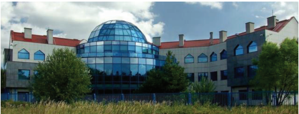
Fig. 1. General view of the CUS building in Psary
