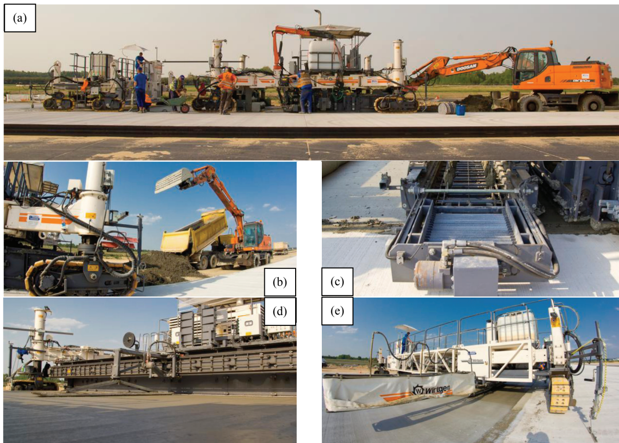
Fig. 6. Construction of a concrete abrasive layer of runway in Pyrzowice, (a) view of 3 parts of band laying machine and excavator, and consecutive concrete laying phases: (b) concrete mix supplied for preliminary spreading with the excavator, (c) element of second part of the spreader placing dowels at the width of the band made, (d) waterproof layer sprinkling system, – view of laying the second band of abrasive surface [own study, on the basis of [17]]
