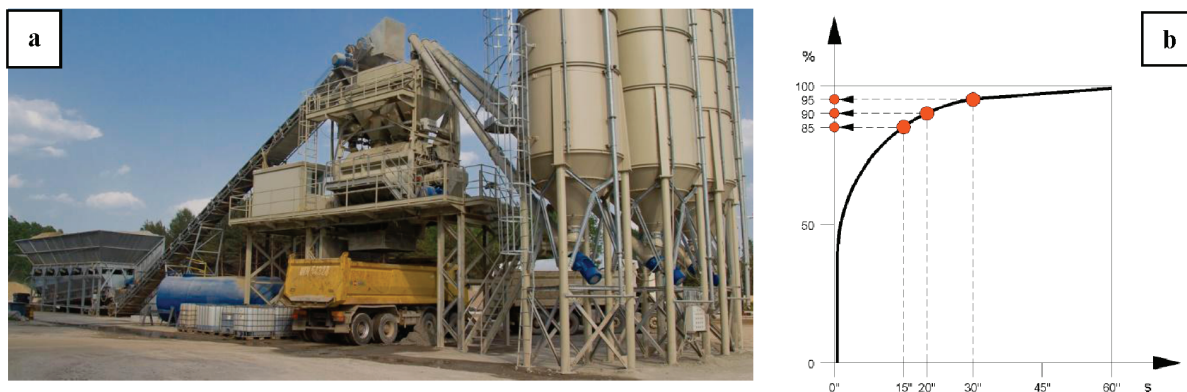
Fig. 5. Concrete plant for the purposes of extending the Katowice-Pyrzowice airport (a) [17], and (b) interdependence of mix homogenisation in %, on the mixing time in seconds, in two-shaft mixers MB [18]
