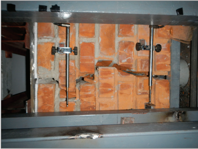
Photo 6. Macrocracks at final stage of force application observed in foundation specimen made of bricks
