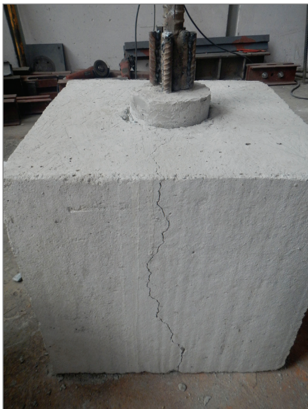
Photo 13. Concrete foundation specimen after the test
